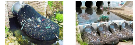
Nets on the drains leading to the dams
