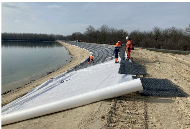
Installation of Renos mattresses for the pilot locker layout - maccaferri
