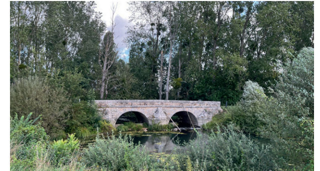
Stone bridge on the road to Port-Saint-Nicolas, Monteuil waterbody
