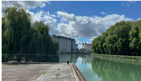
Soufflet malt houses located on the banks of the Seine
