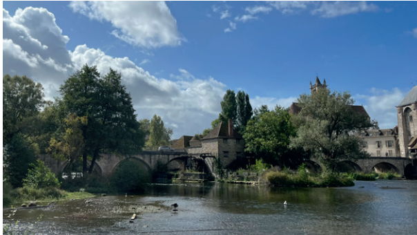
View of the Moret bridge from the banks of the Loing
