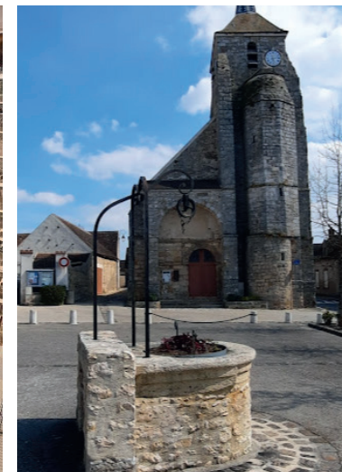
Well at Misy-sur-Yonne.
