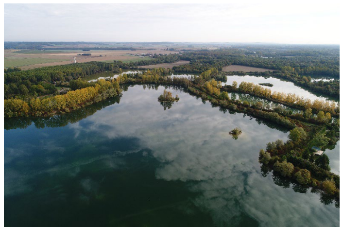
2 The Seine Bassée flood retention basin in Seine-et-Marne, a 360-hectare embanked area designed to protect against major flooding of the River Seine. Source: Seine Grands Lacs
