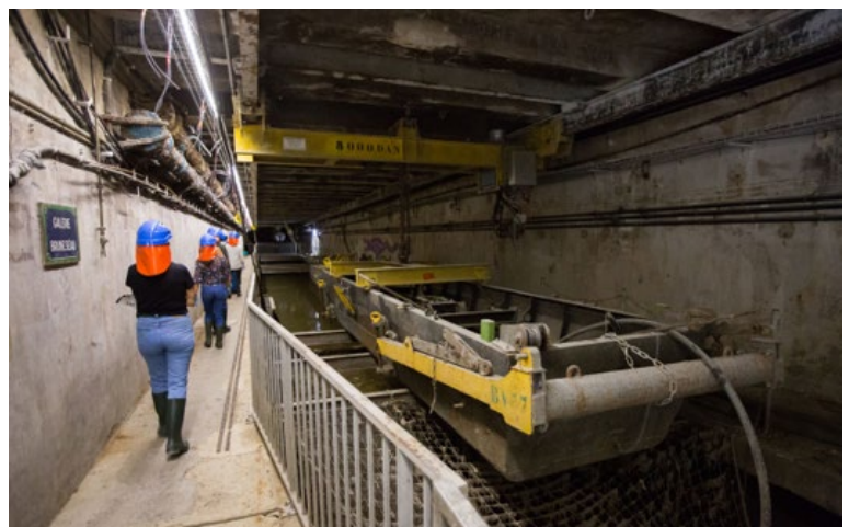
3 A maintenance intervention in the Paris sewers. Source: Jean-Baptiste Gurliat, City of Paris
