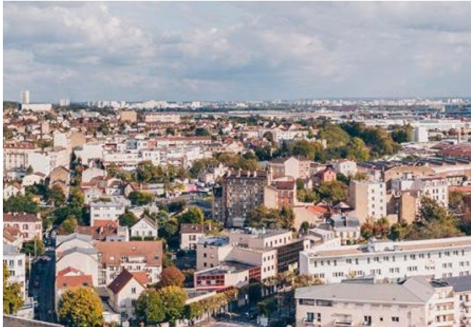
26 Overview of the city centre of Argenteuil. Source: Ville d'Argenteuil
