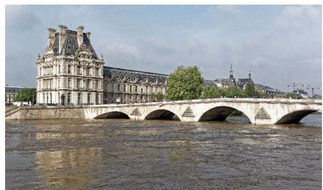
6 The Pont du Carrousel and the Louvre during the 2016 Seine flood. Source: Wikipedia Commons
