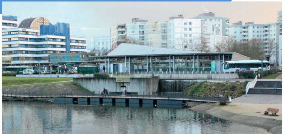
21 Discharge of mine drainage water into Lake CUR, Noisy-le-Grand-Mont-d'Est RER station. Source: Apur (2024)
