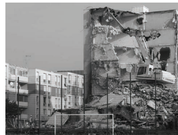
Demolition of the district "Croix-Petit", Cergy 2005
