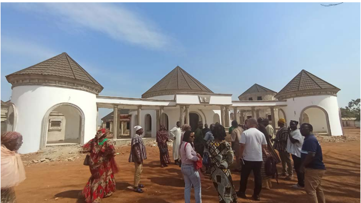
Construction of the new Gbewaa Palace (Source: Les Ateliers, field mission February 2026)
